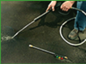
Purging the pump
